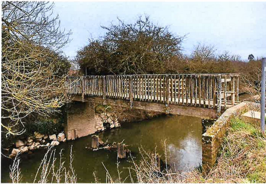
Retention Dam - River Eden from Town Field
