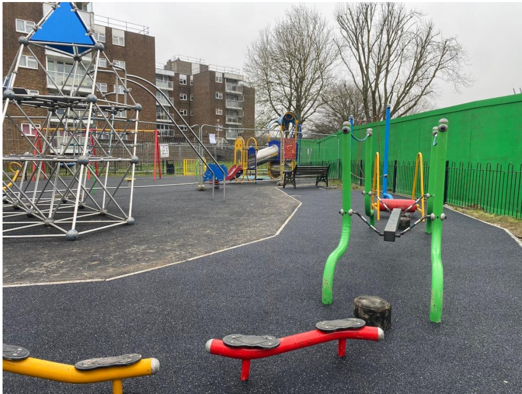
Spitals playground January 2025 – additional wetpour and correction works
